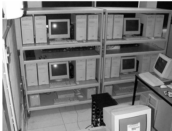
Figure 1: 16-node switched-SCI cluster at Trinity College Dublin.
