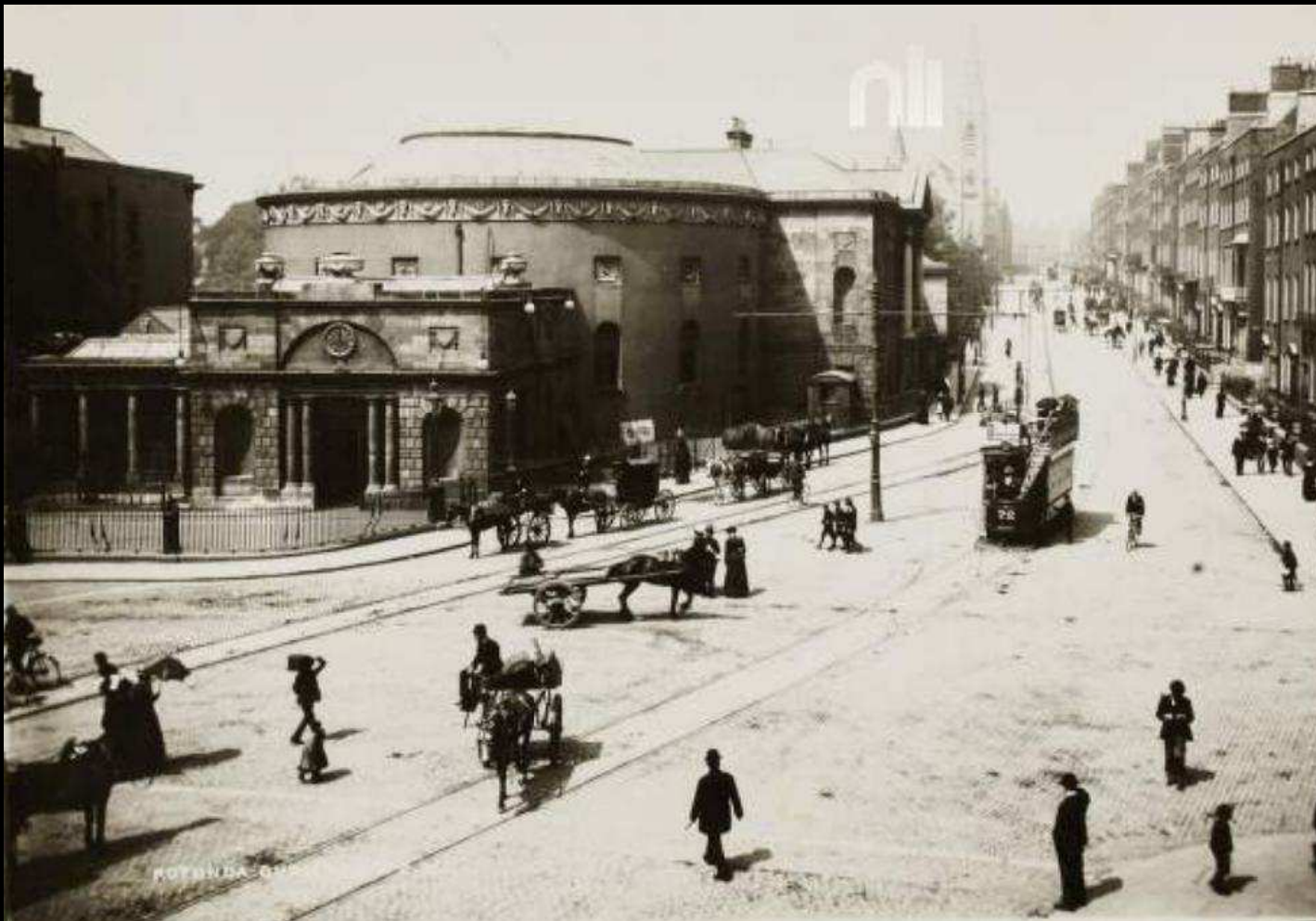
Rotunda Room, Dublin © National Library Ireland
